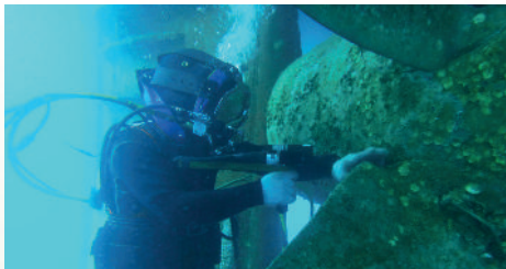
Harbor Star Diving and Marine Maintenance diver inspecting for possible oil leak in shaft seal
